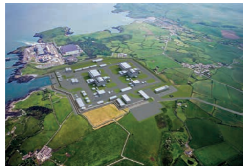
Power systems and equipment
